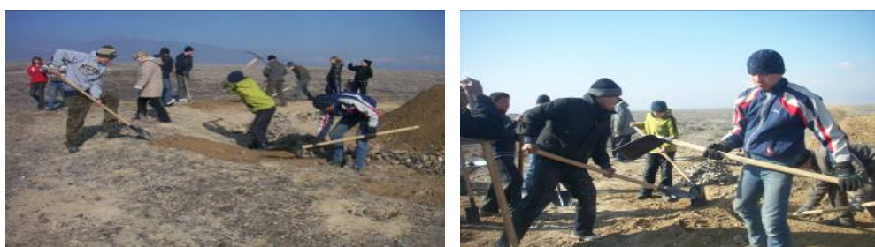
Figure 5 - The work is in full swing
